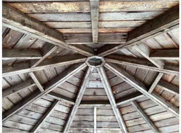
Roof underside overview
