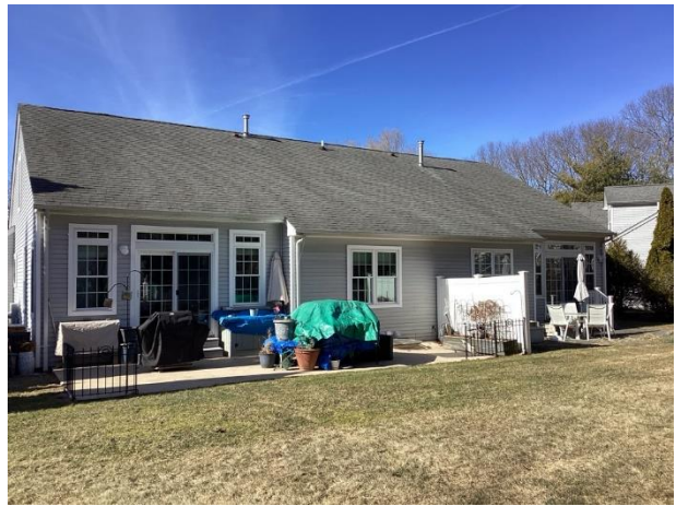
Typical rear elevation overview
