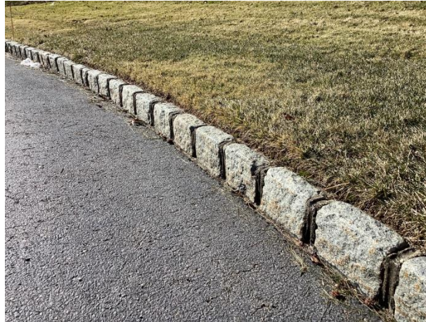
Granite curbs overview
