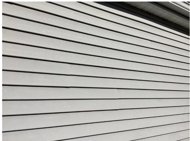
Vinyl siding overview
