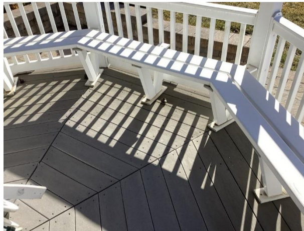
Railings, benches and deck boards overview
