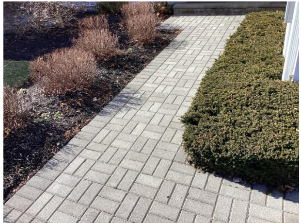
Paver entrance walk overview
