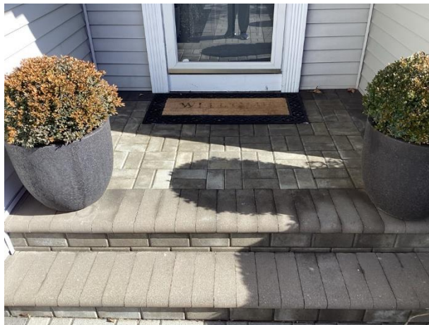
Paver stoop overview
