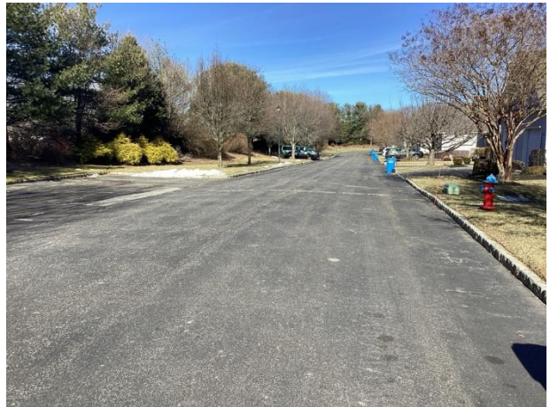
Asphalt pavement street overview
