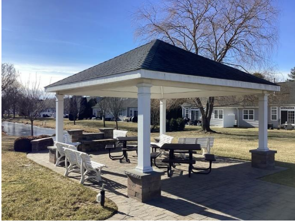
Shade structure overview
