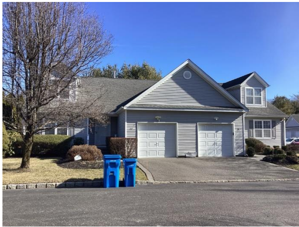
Typical front elevation overview
