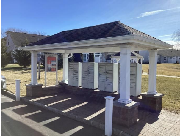
Mailbox station kiosk overview
