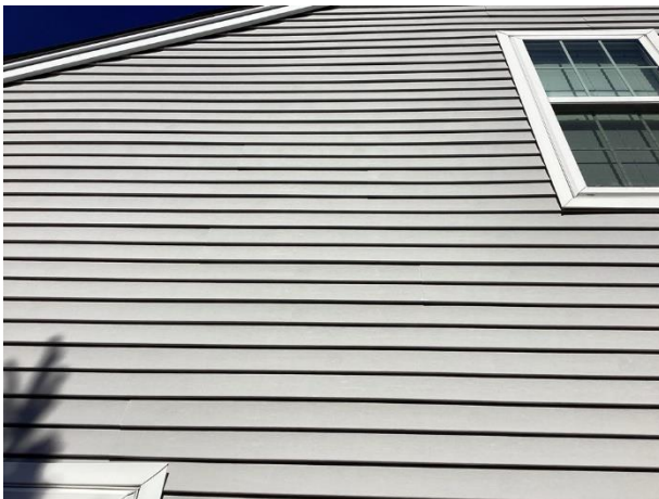
Vinyl siding overview
