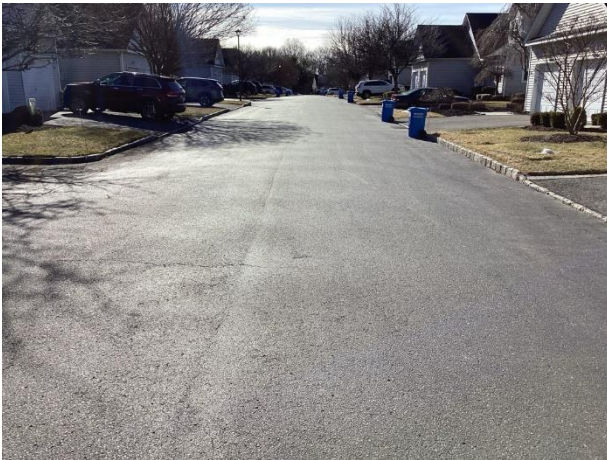
Asphalt pavement street overview
