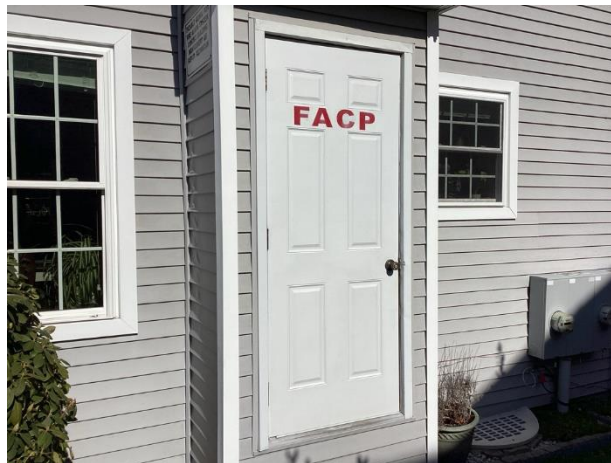
Typical fire control room door overview
