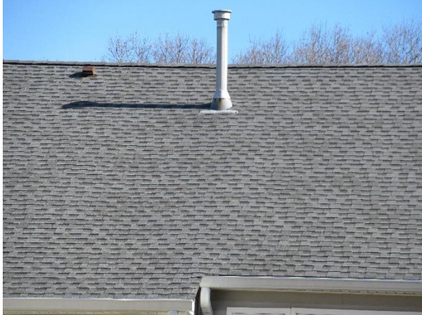
Asphalt shingle roof overview
