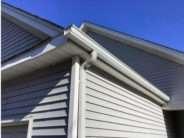
Typical gutter and downspout overview
