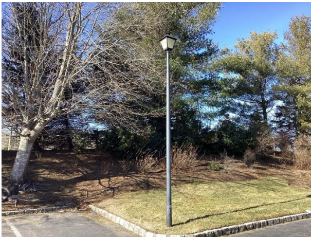
Typical light pole and fixture overview
