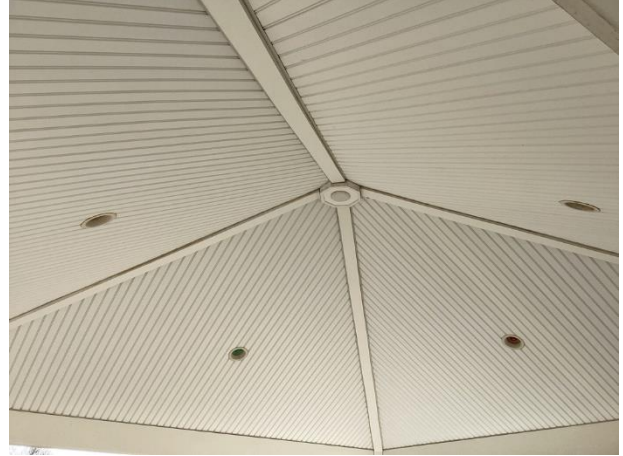
Roof underside overview
