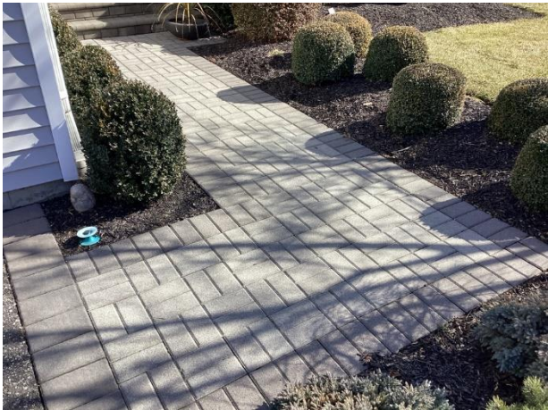
Paver entrance walk overview
